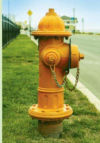
To ensure you receive the highest quality water, Aquarion routinely cleans out the accumulated sediment in all of our water systems. Following a system-wide schedule, we open fire hydrants for a set time to allow the fast-flowing water to flush sediment out of the water mains in the water system.
