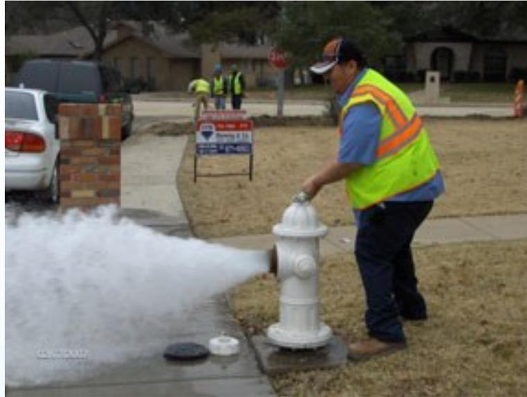
The fall season is typically the time when Aquarion staff flushed water mains. This important maintenance activity removes minerals and sediment that accumulates in water mains, which can cause discolored water. While discolored water is not a health issue, it does reduce the aesthetic quality of water for domestic uses.
