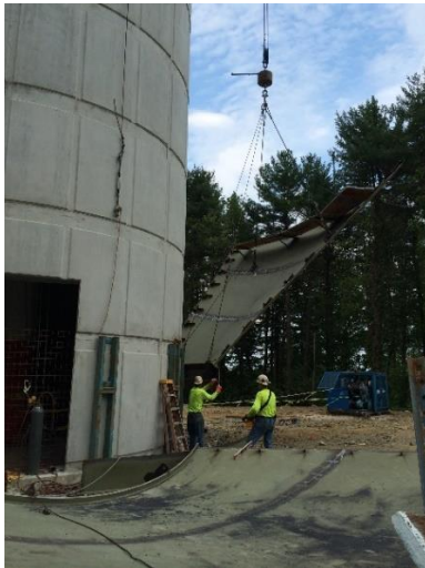
PHOTOS 6-7: Tank Bowl Construction at Ground Level
