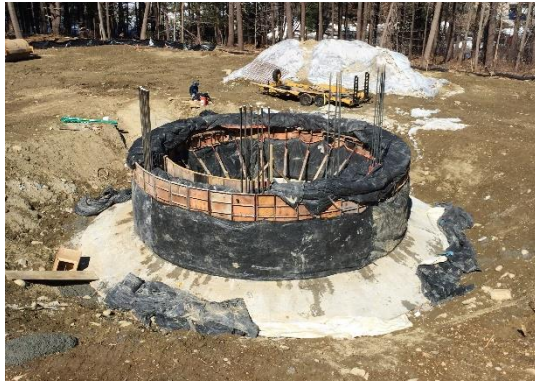
PHOTO 2: Tank Foundation
