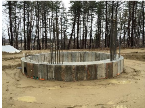
PHOTO 3: Tank Foundation Wall Backfilled
