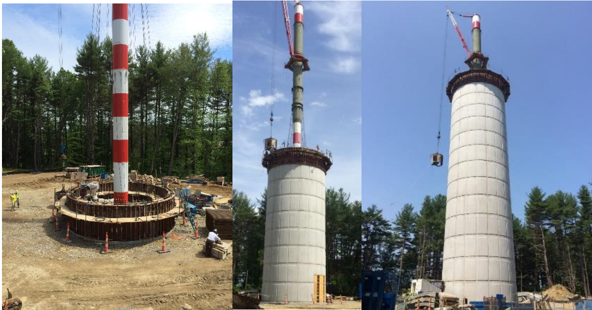
PHOTOS 4-6: Tank Pedestal Construction
