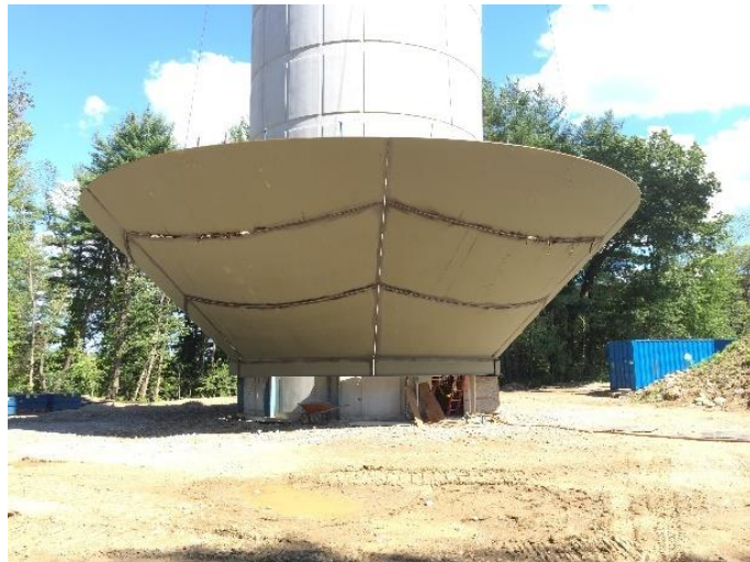
PHOTOS 6-7: Tank Bowl Construction at Ground Level
