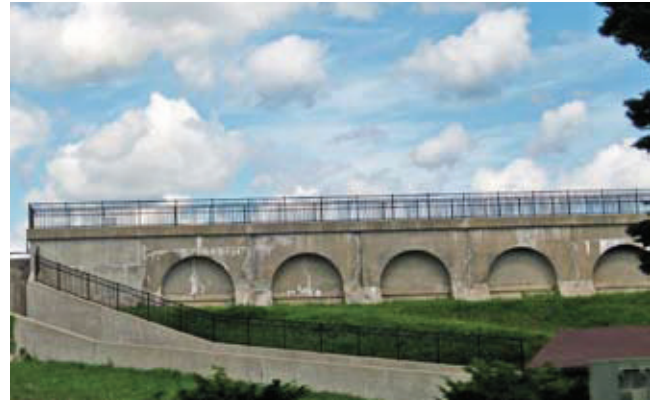
The Trap Falls dam
